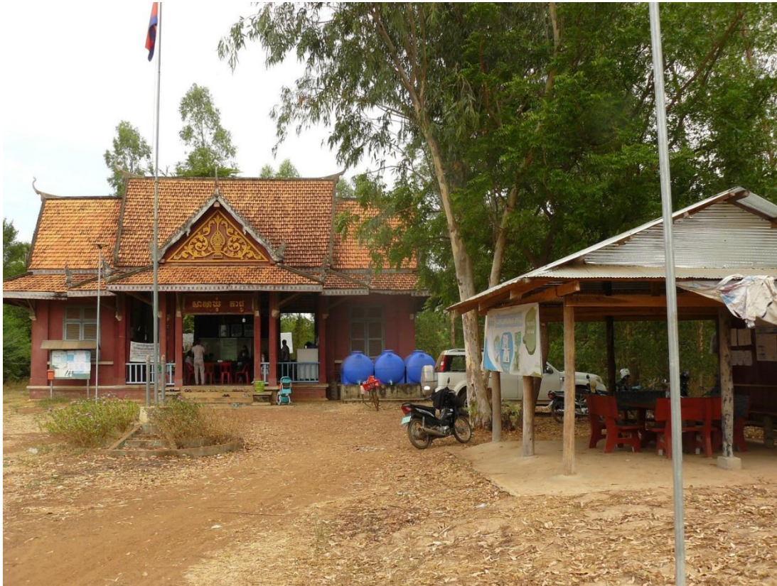
Fig. 5: Typical commune administration building, as constructed under an ADB programme in all six sample provinces.
